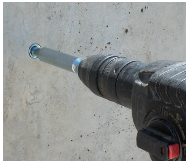
Anchor being set with SDS setting tool.
