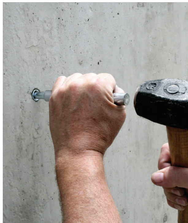
Anchor being set with hand setting tool.
