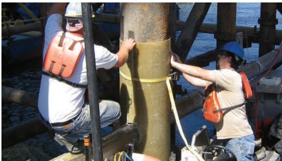
FX-70® structural piling repair and protection system
