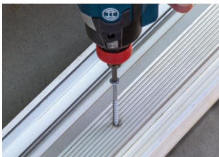
Sliding door track installation
