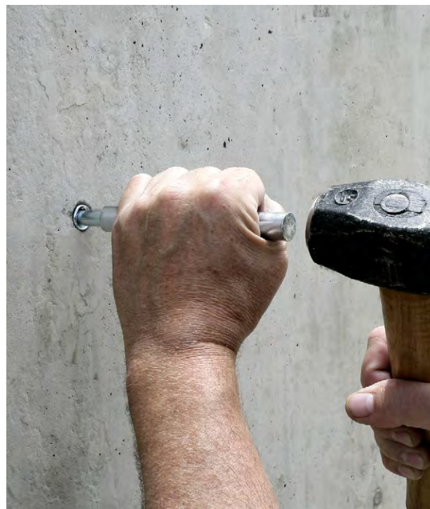
Anchor being set with hand setting tool.
