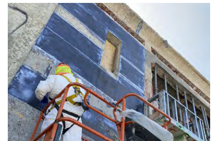
Shearwall Strengthening
