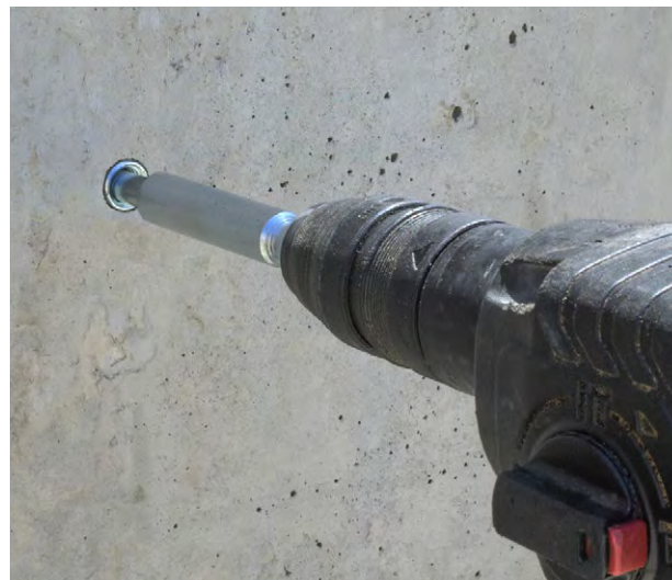
Anchor being set with SDS setting tool.
