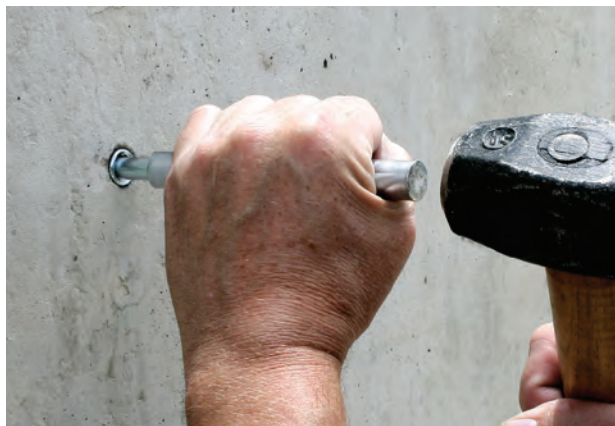
Anchor being set with hand setting tool.
