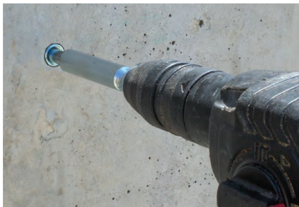
Anchor being set with SDS setting tool.
