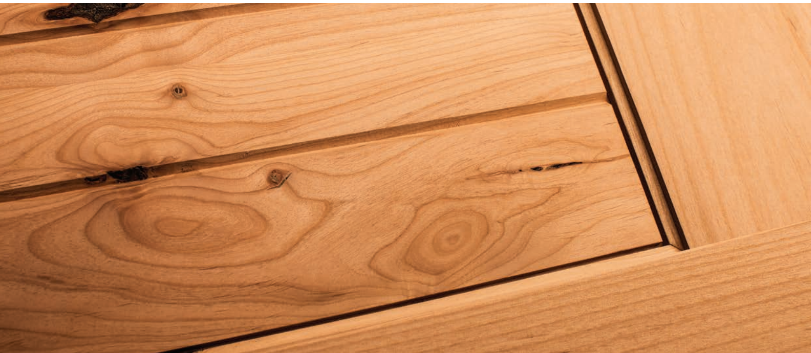
V-Groove Plank Raised Panel, Tapered Sticking
