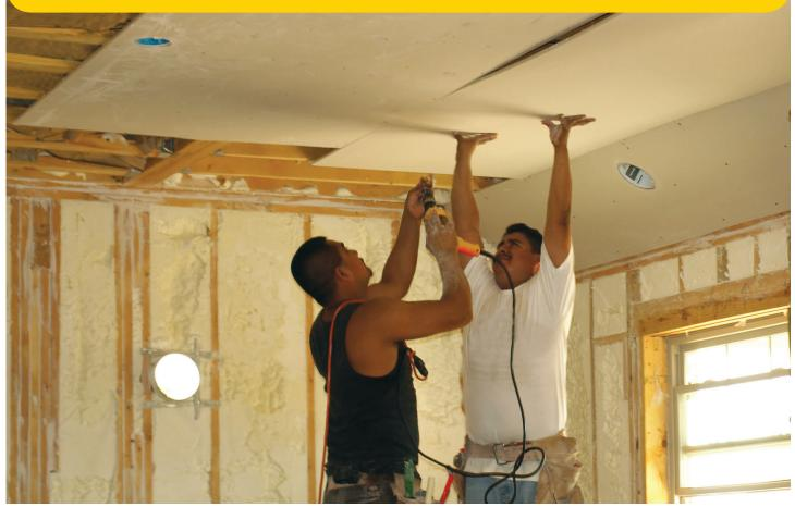
Gypsum board ceilings provide about 3 times longer fire resistance for evacuation -- almost 27 minutes with I-Joists covered by drywall vs. under 10 minutes to subfloor burn-through with any joist assembly that hasn't been drywalled.
