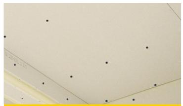
**CEILINGS DRYWALLED WITH GYPSUM,** a natural fire fighter, to BCI® or AJS® joists. Gypsum board ceilings provide about 3 times longer fire resistance than 2x10 joists not covered by gypsum.\*
