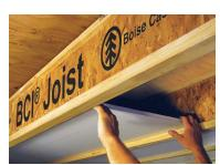
DROP-IN-DRYWALL FIRE PROTECTION with easy access to plumbing, heating and electrical. Uses 12" gypsum — quick and easy to install with no nailing or screwing.
