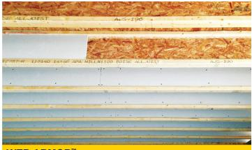
**WEB ARMOR**<sup>™</sup> vertical installation also pairing BCI® or AJS® joists with gypsum drywall – as mentioned above, well known as a famous fire fighter for generations.
