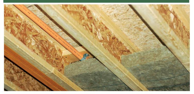
Boise Cascade is now introducing another fire-resistant I-joist solution to increase residential fire protection. This program combines Boise Cascade engineered wood I-joists and mineral wool insulation to insulate better and suppress residential fires for longer periods of time. These products also solve two important code issues – new energy conservation code provisions for insulation in the floor cavity, and new fire resistance code requirements.
