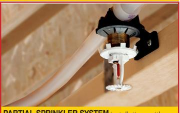
**PARTIAL SPRINKLER SYSTEM** installations with BCI® or AJS® joists, part of a residential cold water system. Could be installed to protect a specific area or hazard even though the rest of the home may not require it.
