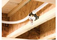
PARTIAL SPRINKLER SYSTEM installed with AJS® or BCI® joists is part of a residential cold water system protecting certain zones of the home.
