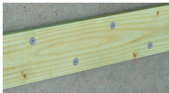
Typical Titen HD Washer Head Deck Ledger Attachment
